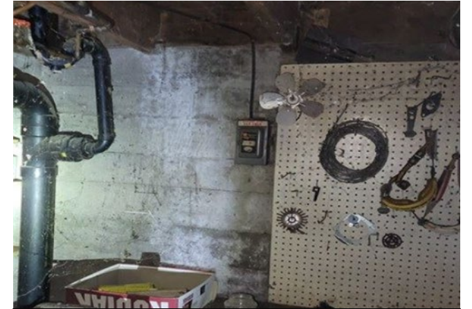
Efflorescence
